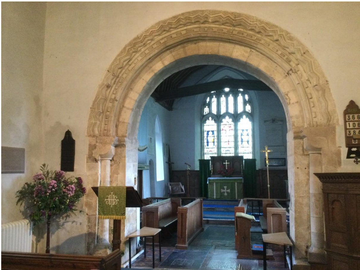
Fig 1 Interior looking east to the chancel arch
